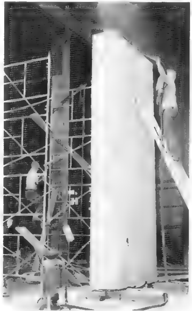
Special scaffolding had to be erected where The Georgia Guidestones were fabricated so that Charles Clamp could sandblast-inscribe over 4,000 letters which were approximately four-inches high on each stone. The languages were chosen because they represent those spoken by a majority of the people in the world.
